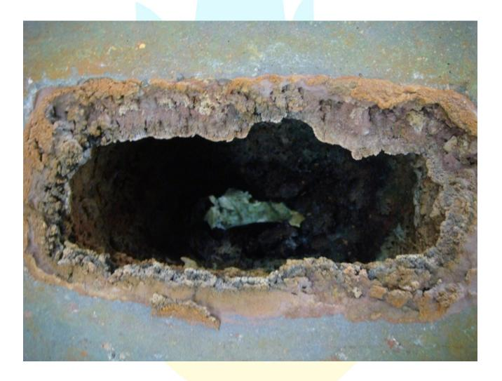
Keep the inside, rear and top lip of the flues clean and free of debris. If the flues remained blocked it's a sure way of destroying the inside of the furnace. It may also buckle the back of the furnace and damage the Burner equipment.
