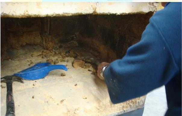
Clean out any loose chippings, build up, broken pots and so on.
